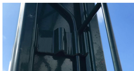
CLIP FIXATION POTEAU/PANNEAU
